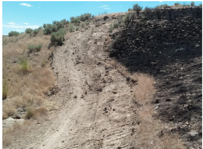
Completed dozer line repair on Martin Fire
